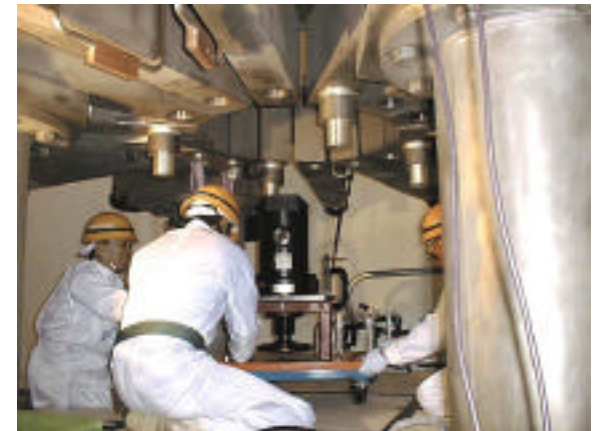
Base structure and tie rods provided by US being assembled at JAERI
