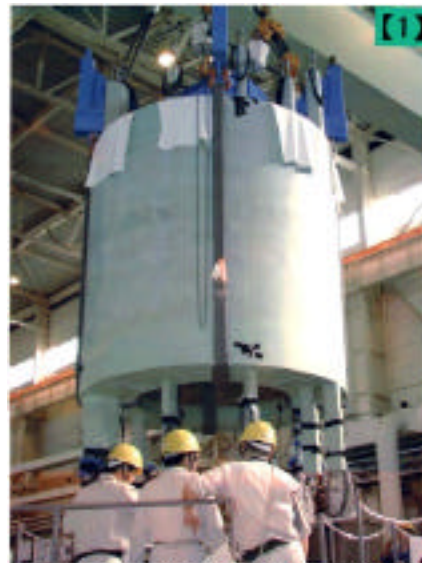
CS Model Coil Inner Module brought above the vacuum tank (June 9, 1999)
